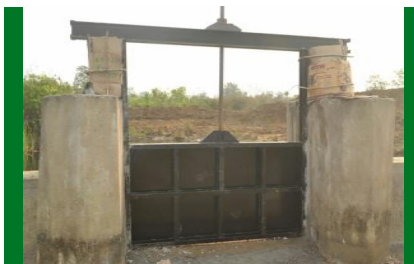
Check dam with percolation pond
