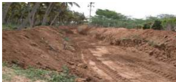
Photo: Channel after excavation
