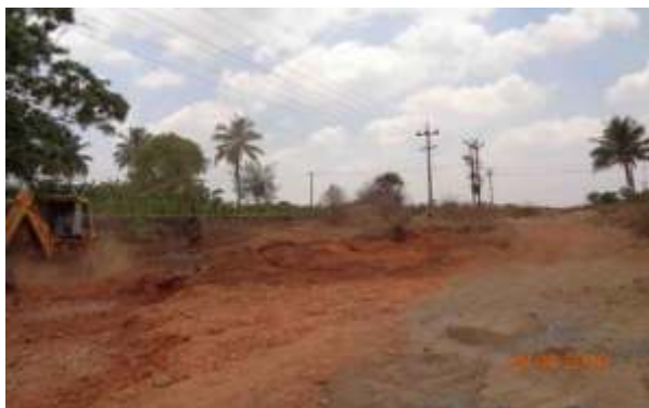
Photo: Site before check dam
