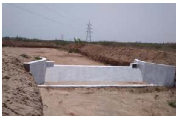
Photo: Check dam cum percolation tank
