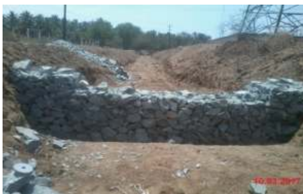
Photo: Gabion Check Dam
