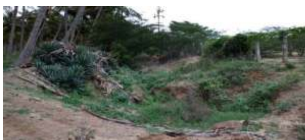
Photo: Channel before excavation
