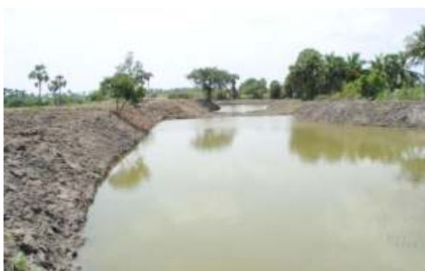
Photo: Flood control by the structure
