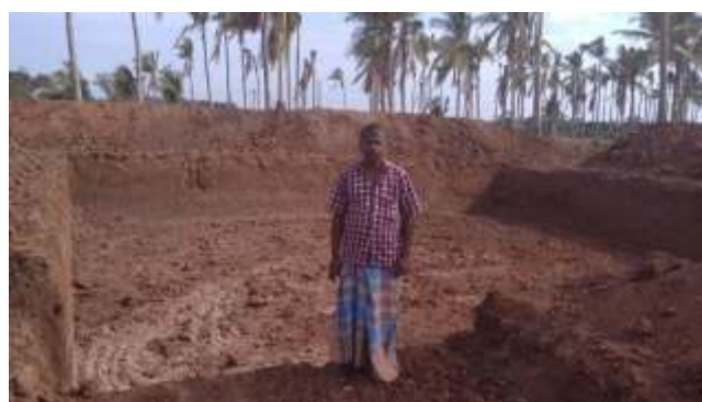
Photo: After farm pond excavated
