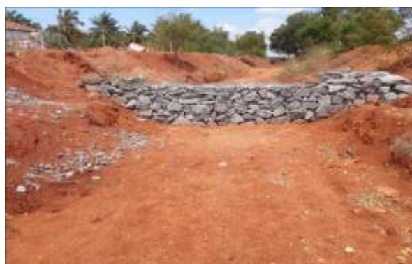
Photo: Gabion check Dam
