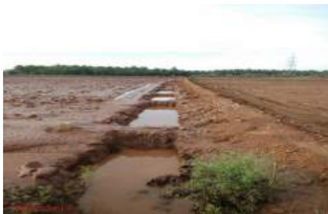
Photo: Water absorption Trench and field bund
