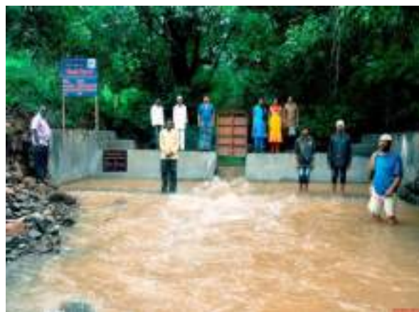
Photo: After construction of check dam
