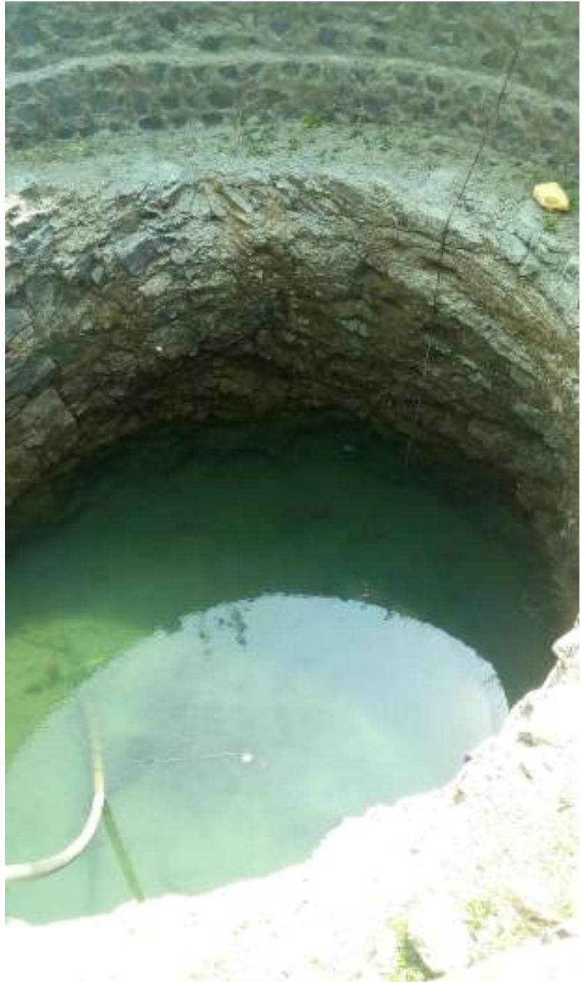
One of the observation well in the project area
