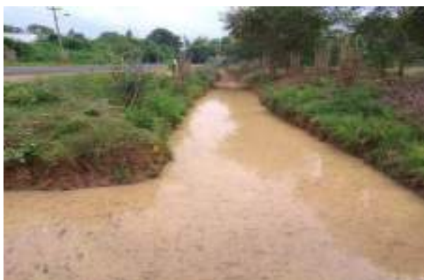
Photo: Water flow in cleared channel
