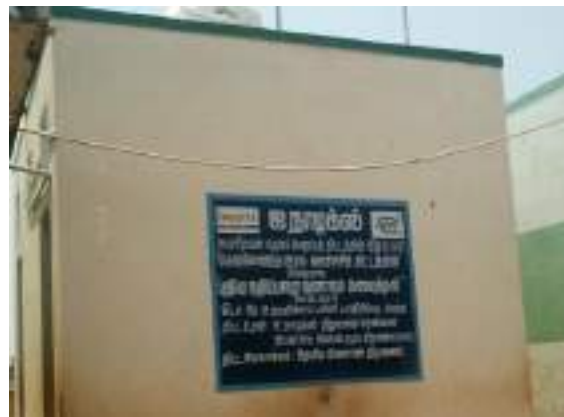
Photo: Newly built sanitation complex in a village school
