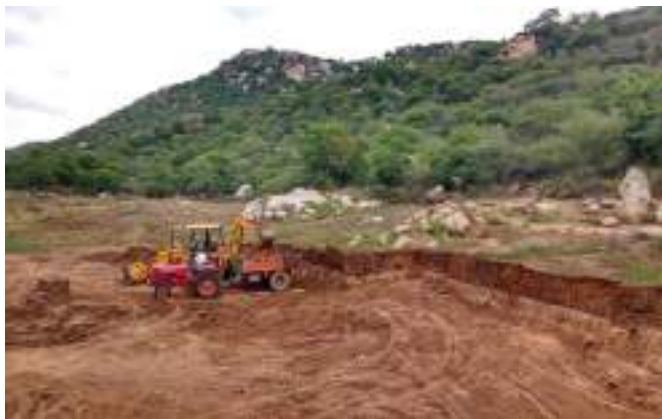
Photo: Desilting of lake during project
