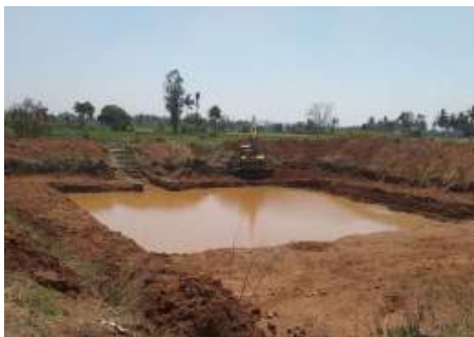
Photo: Percolation pond of Melpennathur after construction
